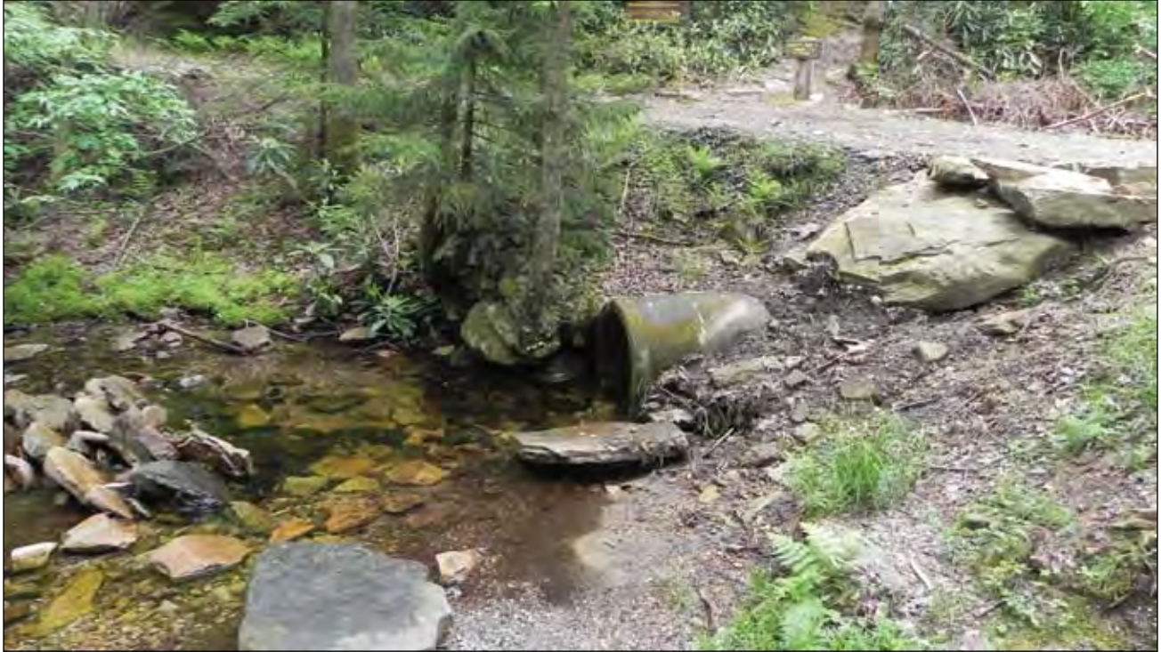
An old culvert. Land managers are beginning to replace culverts like this one with larger culverts designed to accommodate larger peak flows and allow the passage of aquatic organisms. Photo by Patricia Butler, NIACS and Michigan Tech, used with permission.
